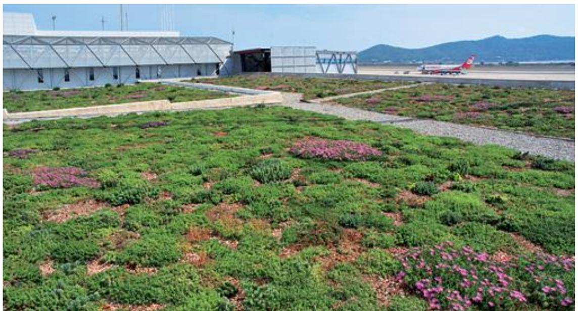
*Figure 2-4: Extensive Green Roof*
