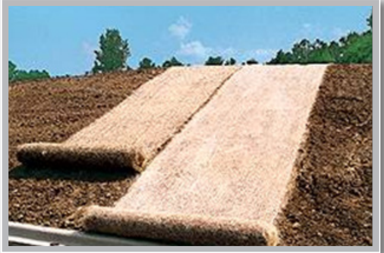
Figure 3.3: Application of an erosion blanket 1
