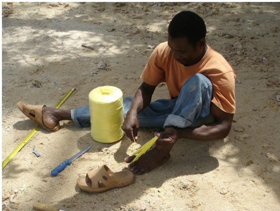
Fig. 19 Cutting tie tie into required lengths
