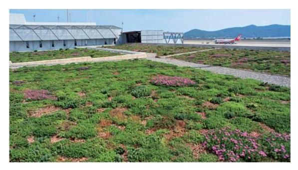
Figure 2-4: Extensive Green Roof
