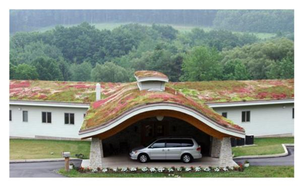
Figure 2-3: Green roof on flat and pitched roofs
