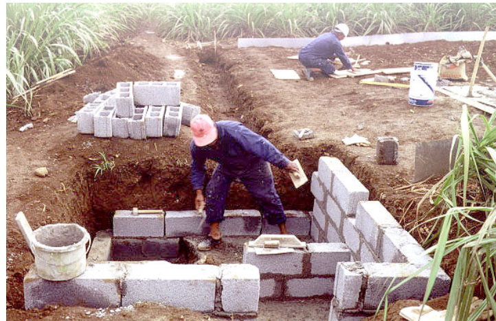
Fig 4. Construction of pit for installing collecting devices
