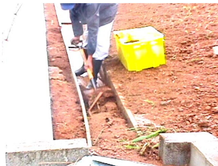
Fig 8. Collecting eroded soil from troughs
