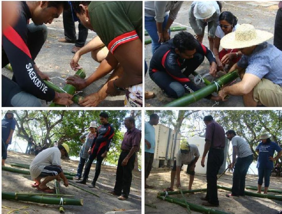
Fig. 12b Construction of bamboo raft. Note also the fixing of side poles to strengthen the raft
