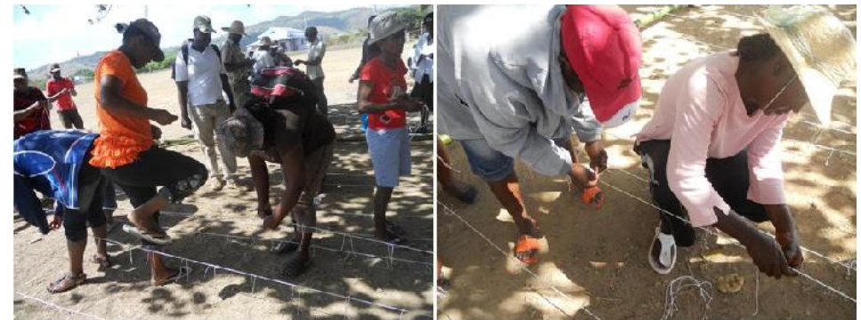
Fig. 30b Preparation of ropes and tying ropes on the bamboo raft
