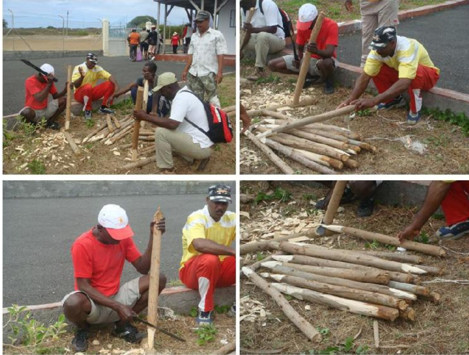
Fig. 34d The wooden pegs preparation group; Sharpening the pegs
