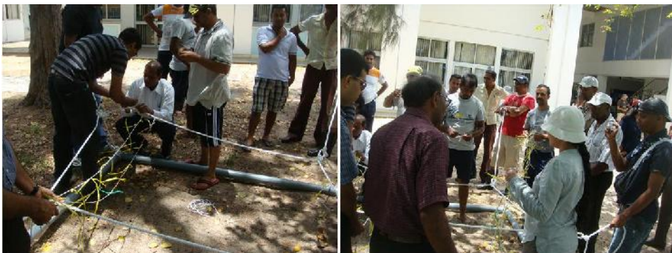
Fig. 13c Attaching lines (4mm ropes) on the thick rope
