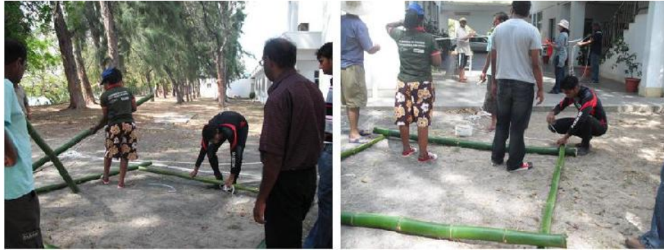
Fig. 12a Assembling bamboo poles for construction of a raft
