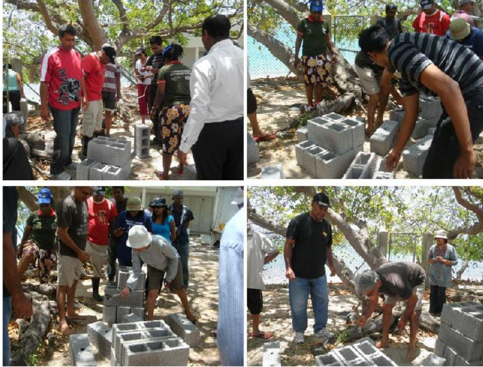
Fig. 15a Preparing the anchors made of cement blocks
