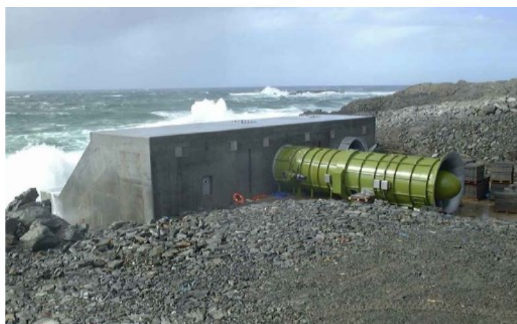
Figure 134: Turbo machinery of the Limpet prior to construction of the main building
